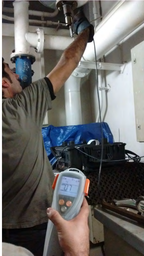
Figure 18. Diesel auxiliary engines emissions measurements.
