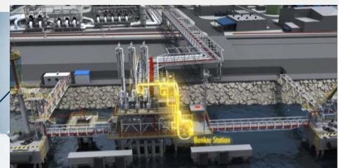
Adaptation for LNG bunkering/small scale services in REGASIFICATION PLANT OF SAGUNTO
