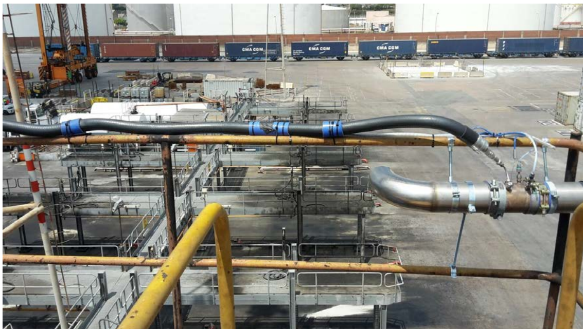
Figure 6. Bundle of heated gas sampling, pressure and temperature lines tied to the railing
