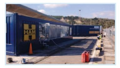
This EPT1 sub-activity pilot aims decentralisation and autonomous power supply of auxiliary engines of a ro-ro ferry in the port. Electricity is generated by a gas engine on the wharf. Tests will be carried out in the ports of Barcelona, Vigo and Tenerife.
